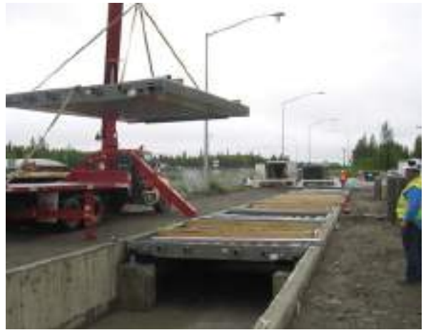
A pit-style scale is placed in an excavated foundation, flush with the ground
