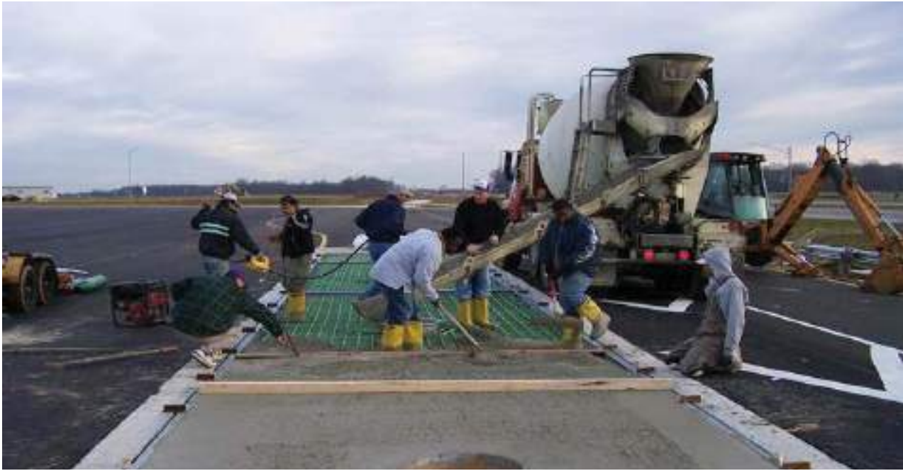
Concrete is poured into the deck of a concrete weighbridge at installation
