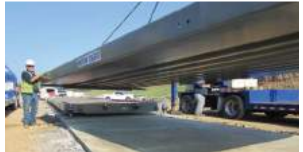
The weighbridge modules are placed into the foundation
