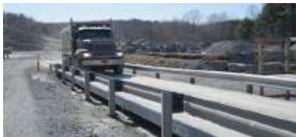
These stand-alone guiderails are planted in the ground alongside the scale to offer added strength and prevent trucks from driving off the side of the scale
