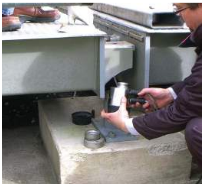
Periodically check load cells, receivers and other critical parts for wear
