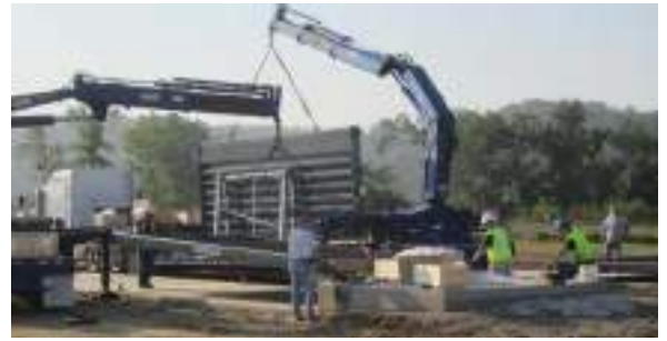
These scale delivery trucks are equipped with on-board cranes used to lift and place the weighbridge modules into the scale foundation
