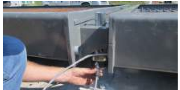
Load cell cables are routed through the scale and attached to the load cells
