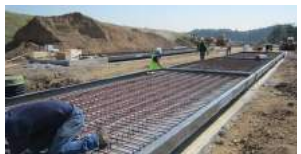
This scale is nearly ready for concrete to be poured into the deck modules
