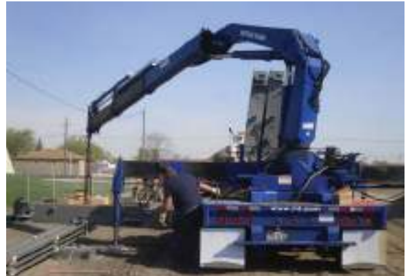
Piecing together a portable frame truck scale on a prepared compacted soil site
