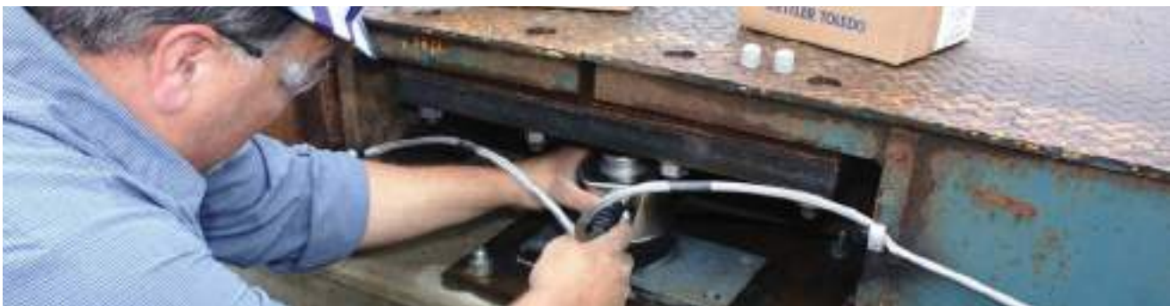
Upgrading an existing weighbridge by installing a new load cell system enhances the scale's accuracy and reliability
