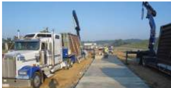
Specially designed delivery trucks are able to transport the weighbridge modules upright
