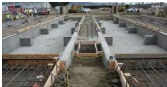
Foundation preparation can take place prior to the scale components arriving on site
