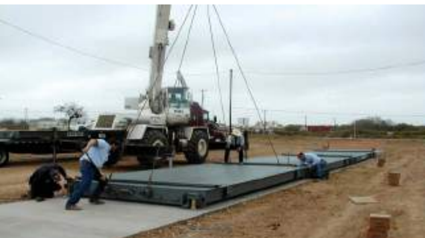
A steel deck weighbridge is installed
