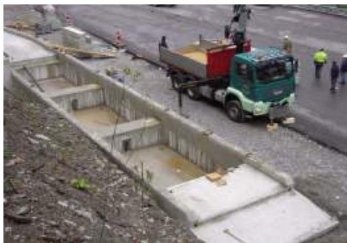
The scale foundation should include adequate approaches that comply with local regulations
