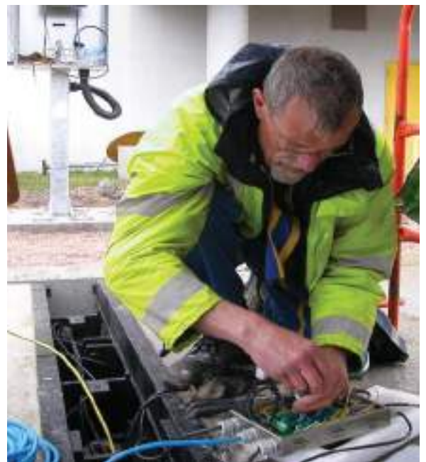
A technician tests load cell cable connections inside a junction box
