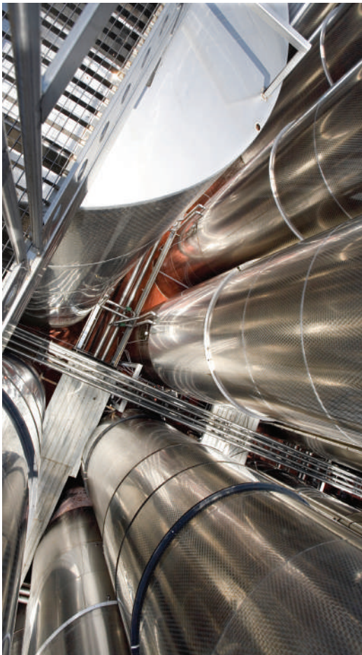
Silo, Tank and Hopper
